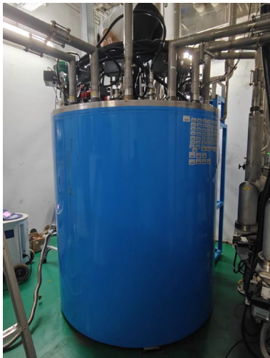
Hydrogen Loop(1.5 MPa@18~21K)
