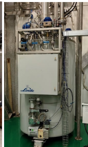
Helium Refrigerator(2.2kW@20K)
