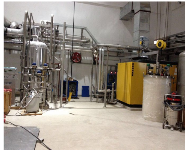
Helium Refrigerator(2.2kW@20K)
