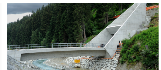
Road access at top Train platform at bottom
