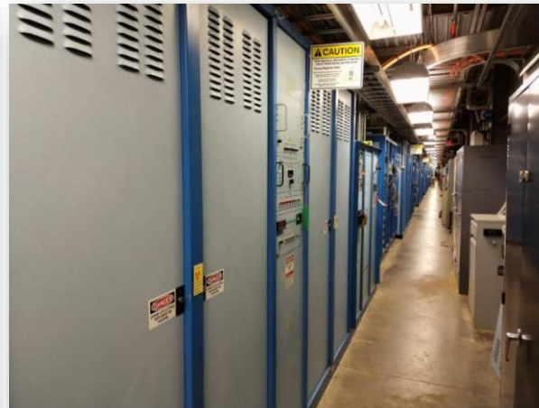
418 Klystrons for 52.25 Cryomodules
