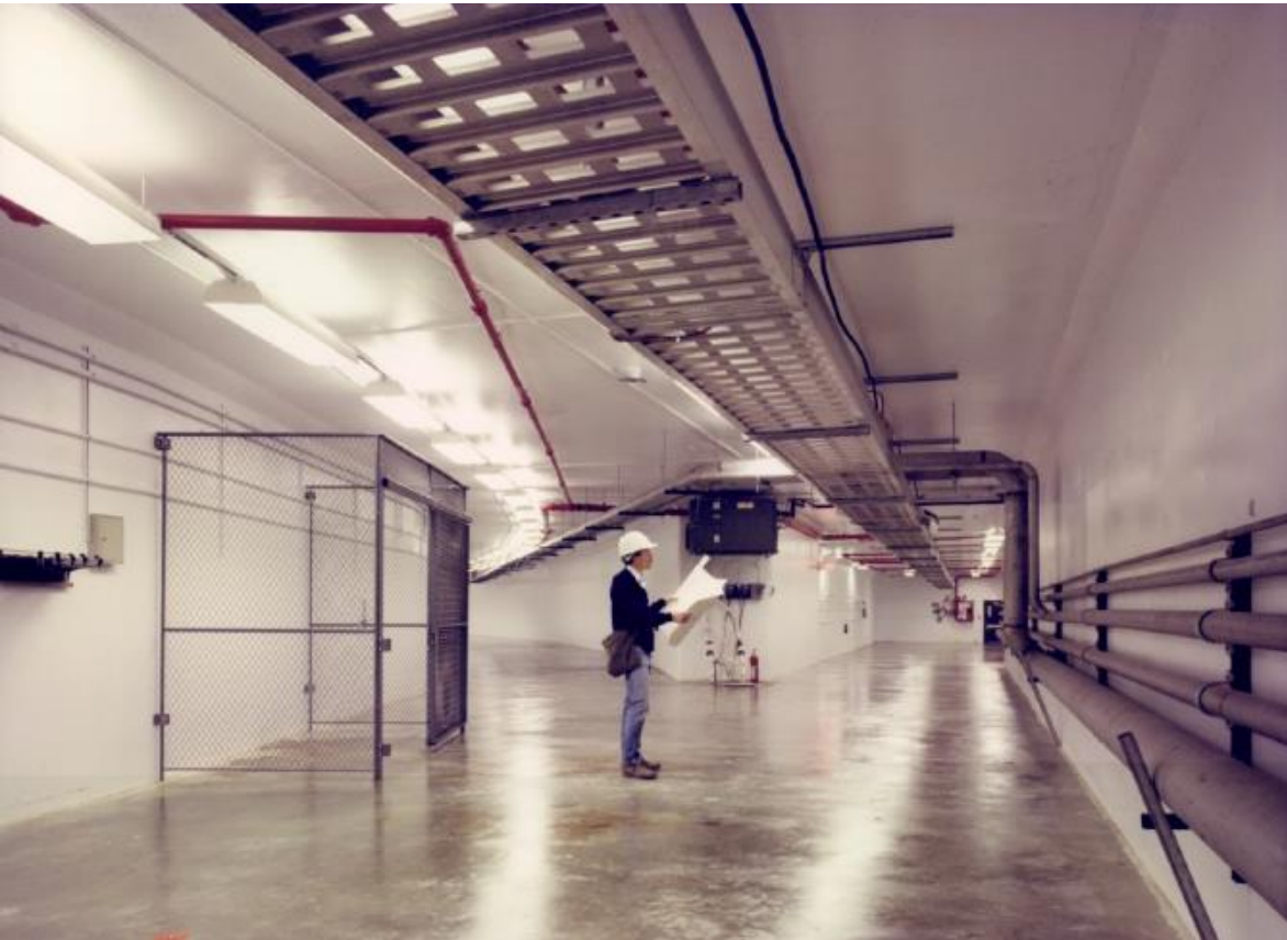
Tunnels before hardware installations
