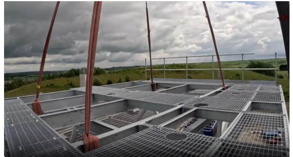
The new coolers being installed
