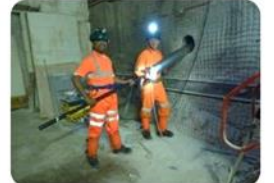
Bore hole detector installation
