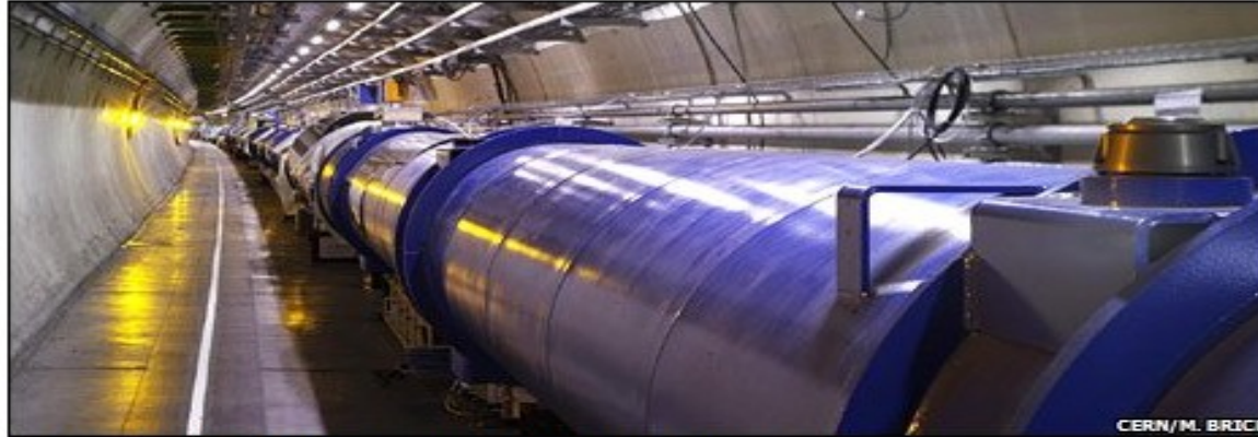
Superconducting magnets are cooled down using liquid helium
