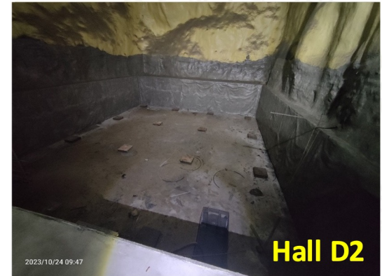
Excavation of Experiment pit
