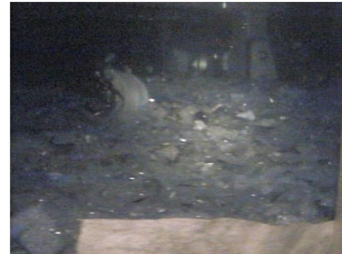
Glass debris at the bottom of tank 29
