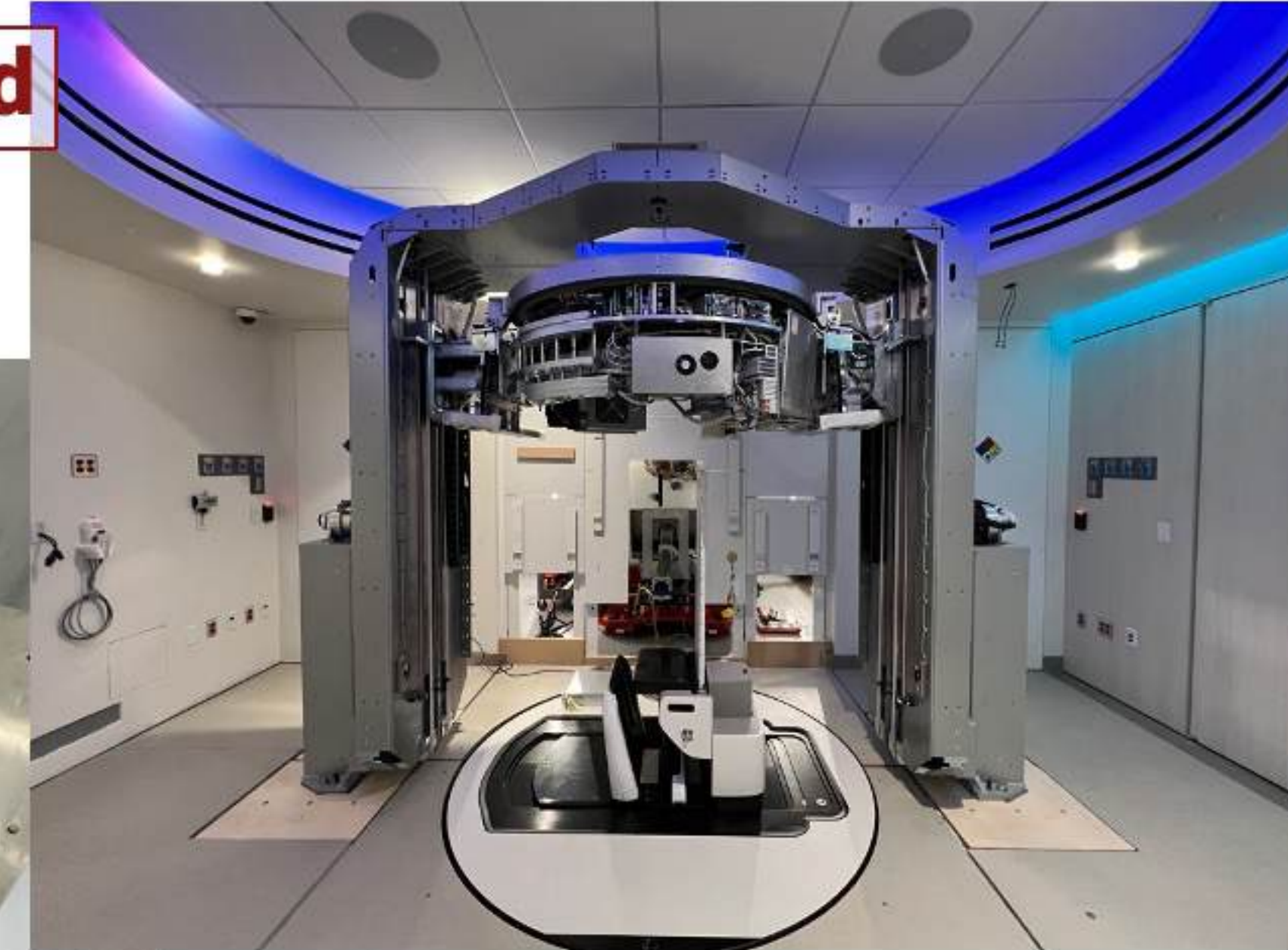
Installation nearly complete
