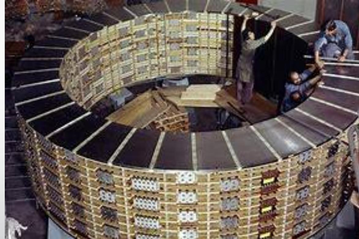
Big European Bubble chamber : Use cryostabilised superconducting coils to generate magnetic fields of up to 3.5T. Largest at the time, boasting a 3m diameter
