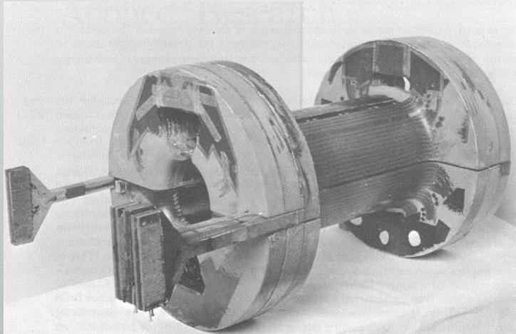
AC3 Magnet prototype produced by RAL (1971)
