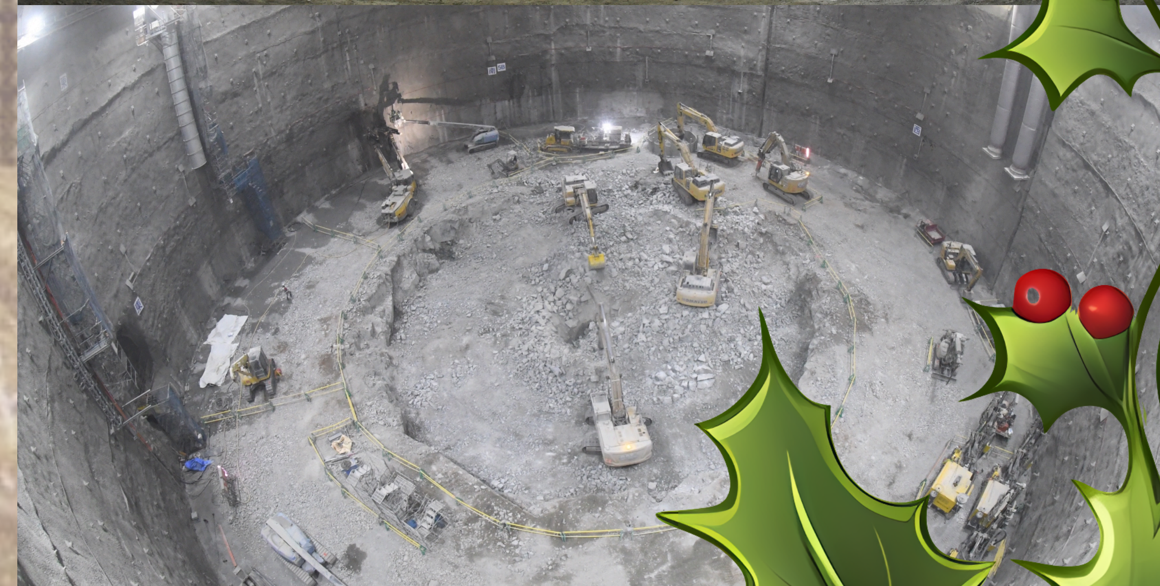
Oct. 3, 2023 Completion of the dome (dia. 69 m, height 21 m, ~1 Super-k)
