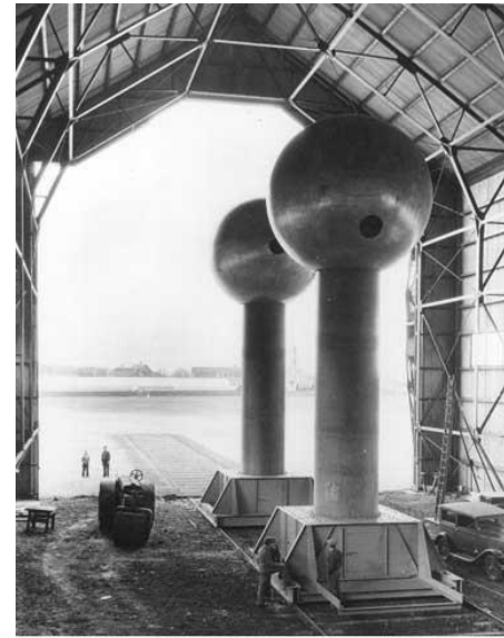
THE GENERATOR IN THE HANGAR AT ROUND HILL ©MIT Museum. All rights reserved.
