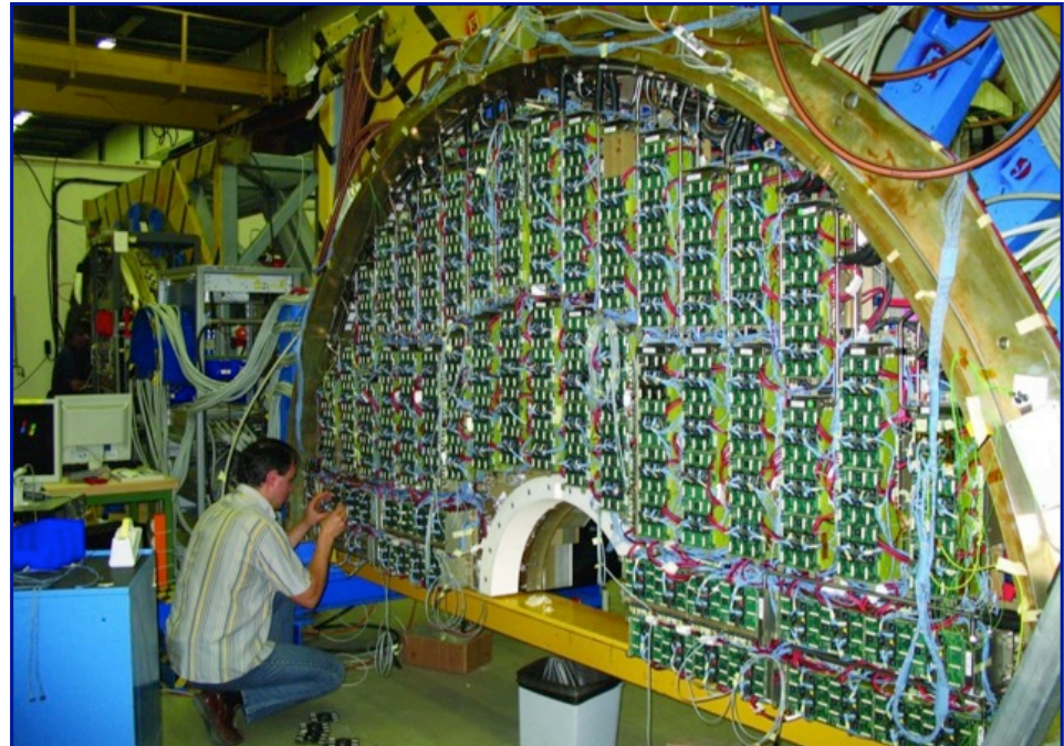
Installation of readout electronics
