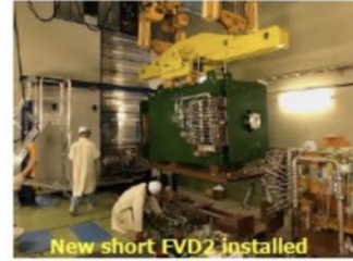
New short FVD2 installed
