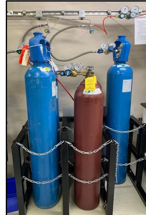
Aged gas cylinders (CO 2 , N 2 , O 2 ) for a minimum of one month
