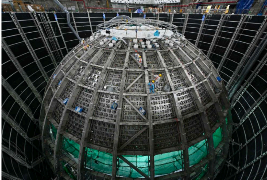
PMT installation, June 2023
